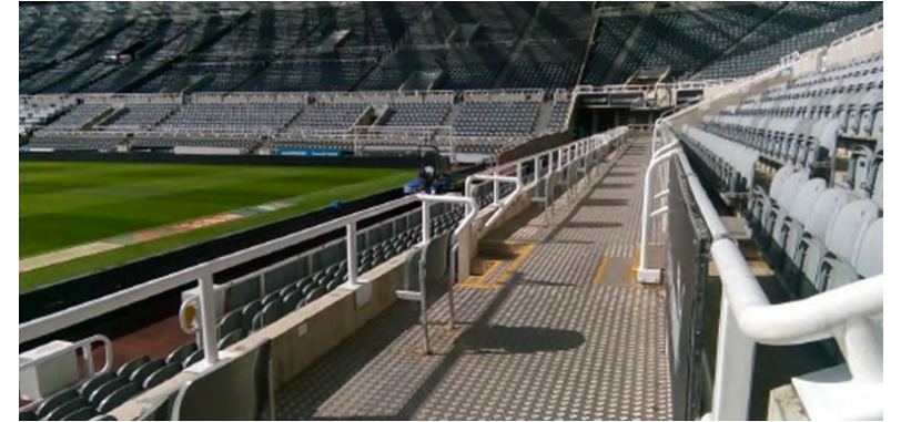
Leazes (North) stand viewing area
